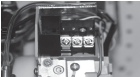
Fig. 9 Power Terminal Block (Indoor Unit)
